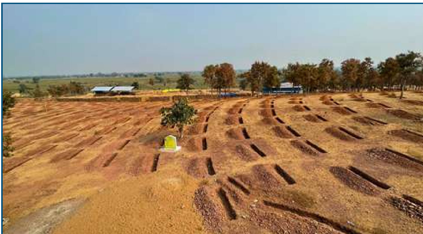
After Intervention work of contour trench
