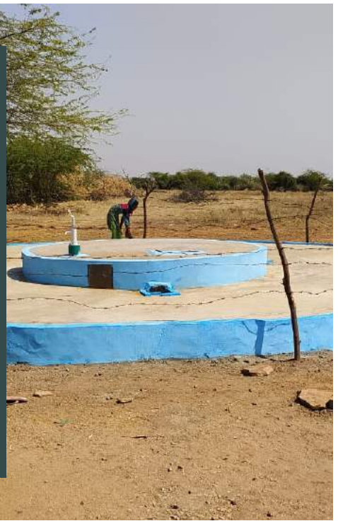
Rain Water Harvesting Structure Tank
