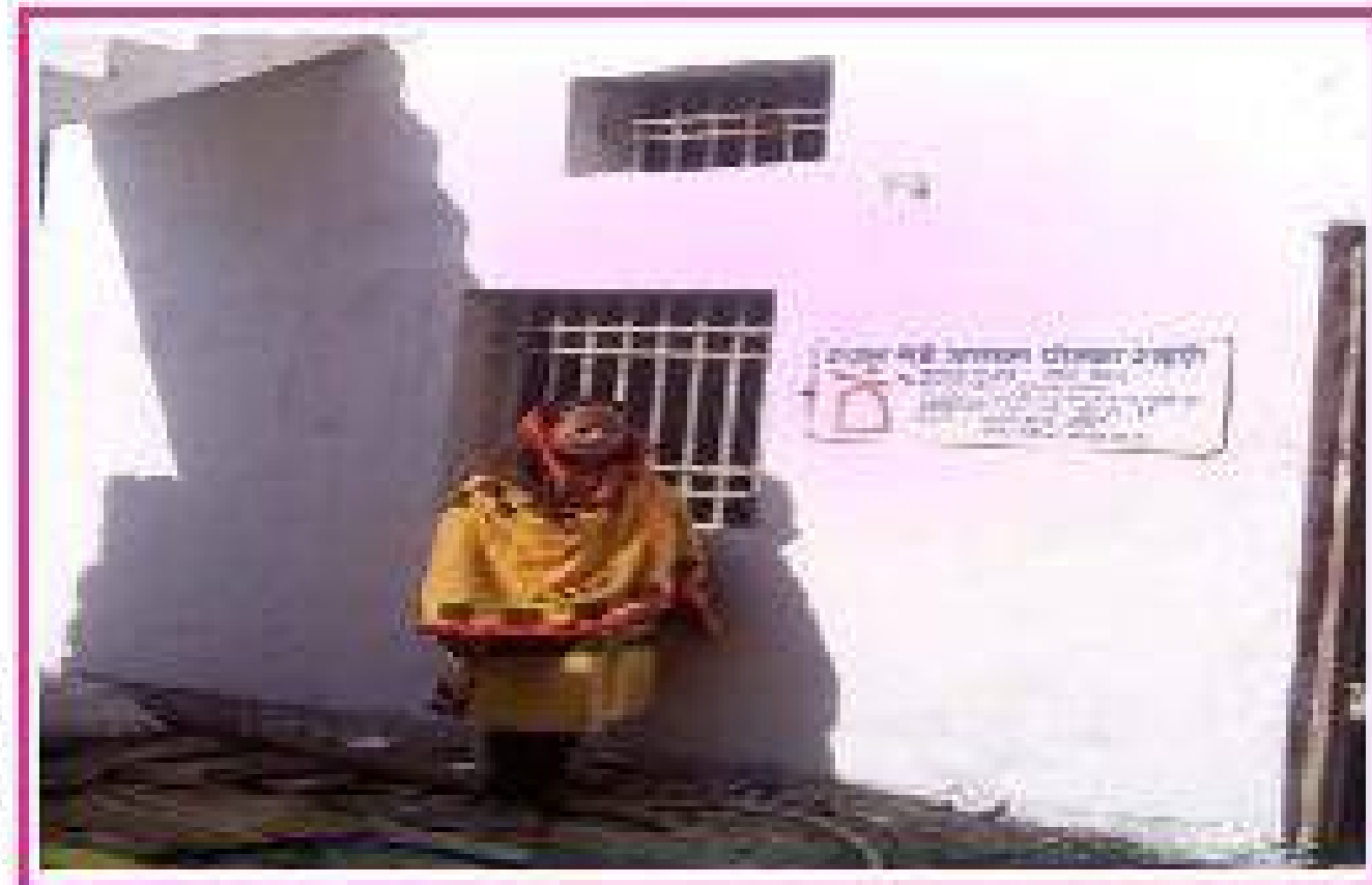
Roushan Niha Stands At Her Newly Constructed (Pradhan Mantri Awas Yojna) PMAY House
